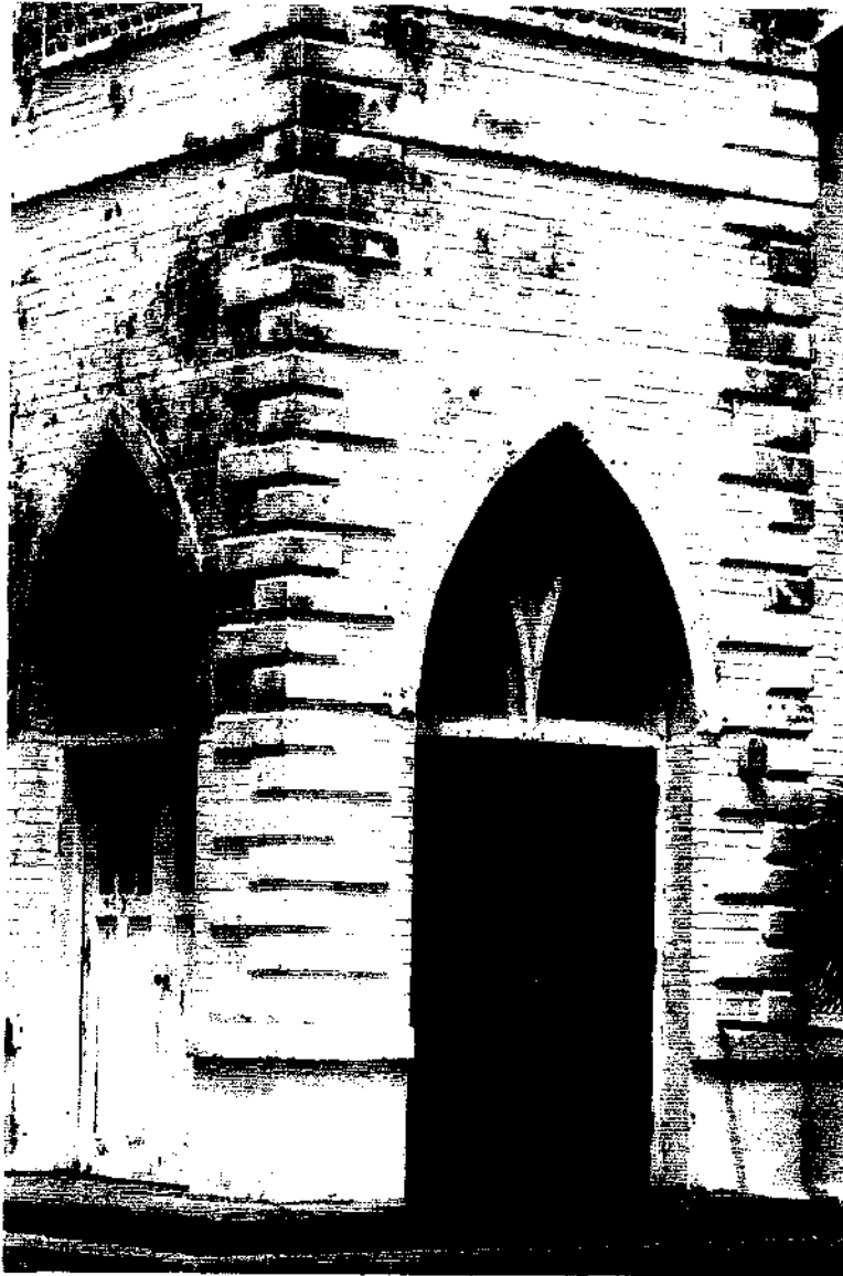
Fig. 8.21 223 Truman Avenue Quoining of Bethel AME Church Bahama Village, Key West, Florida Construction Date: 1925 (older building, in a more desirable location, was built in 1870 and then burned in 1921) Photo by Astrid Whidden Year Taken: 2006
